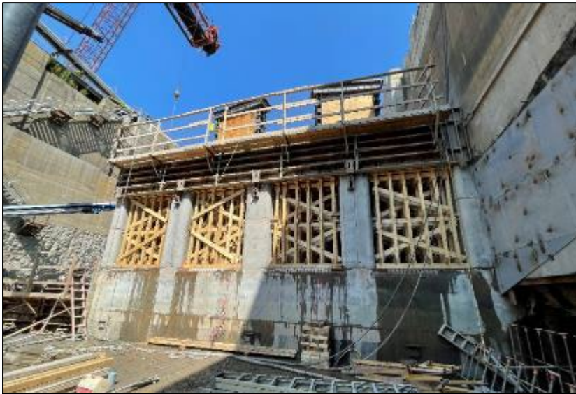
Charleroi River Chamber – U/S Miter & Filling Sill
